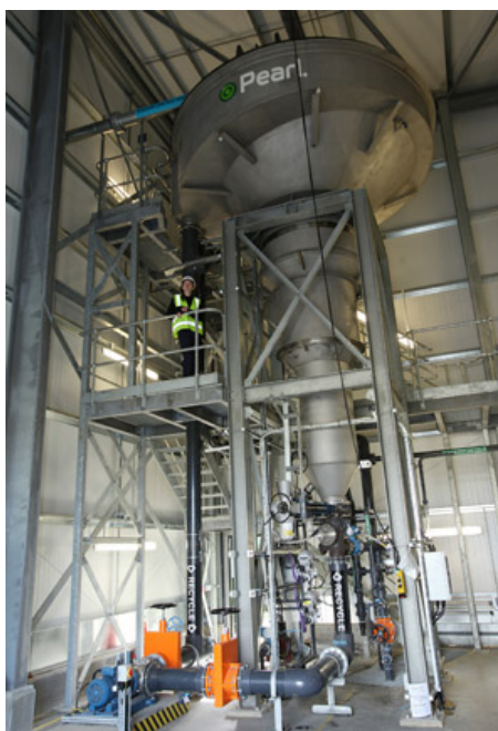
The Ostara Pearl® Nutrient Recovery unit at Thames Water's Slough sewage works
