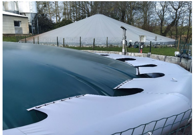
Couiclang pig farm site visit: covered manure storage with biogas collection
