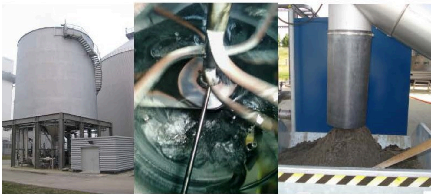
Struvite washing installation
