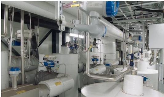
OxyPower HTC™ simplifies both nitrogen and phosphorus recovery. Nitrogen is extracted from the separated nitrogen-rich wet oxidized process water by ammonia stripping. Up to 60% of the nitrogen in the sludge is separated as ammonium sulphate.
